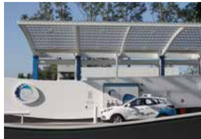
Air Liquide hydrogen charging station in Rotterdam
